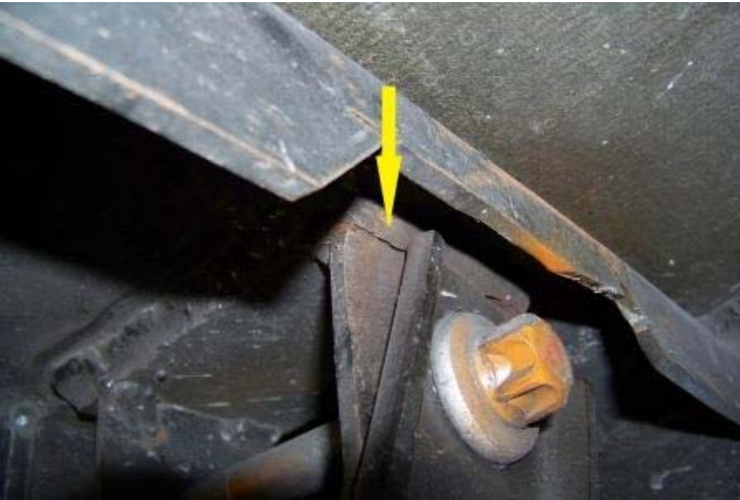
BOTH REAR SPRING HANGER WELDS ARE CRACKING (1,882 TEST MILES)
