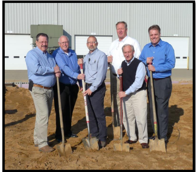
The ARBOC management team breaking ground on the new addition. From left to right: Don Roberts, Mike Skibbe, Blain Hite, Robb Ledbetter, Del Herr, Bill Fay
